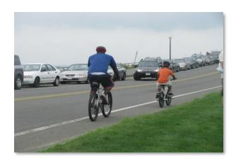
**Striped Bike Lane-**Exclusive use area for cyclists which is adjacent to the outside travel lane. Typically four to five ft. in width, extra protection can be provided by adding
