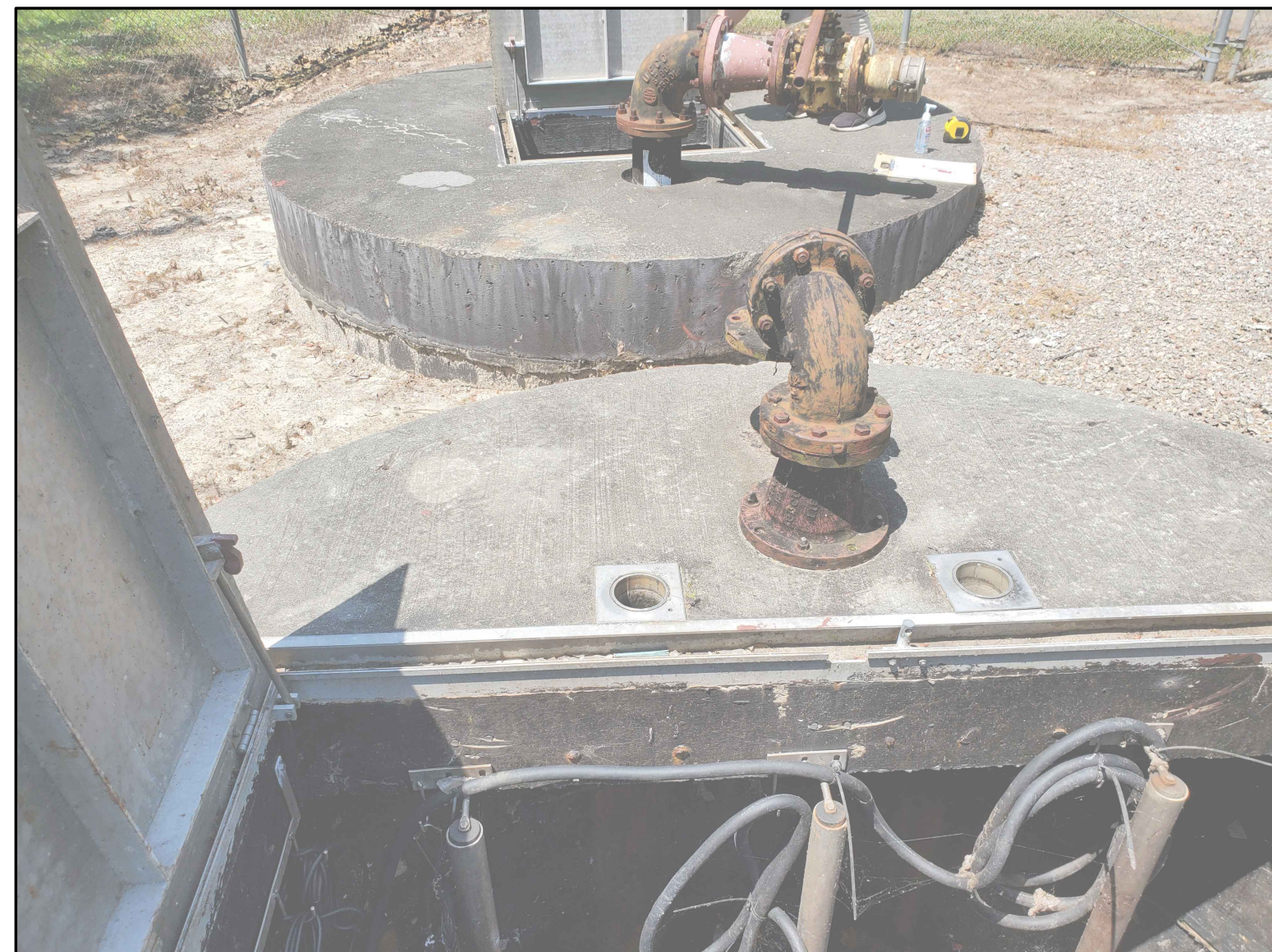
PHOTO-6 LOOKING SOUTHWEST FROM WET WELL TO VALVE VAULT
