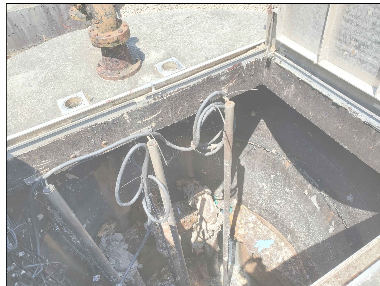
PHOTO-7 LOOKING DOWN IN WET WELL
