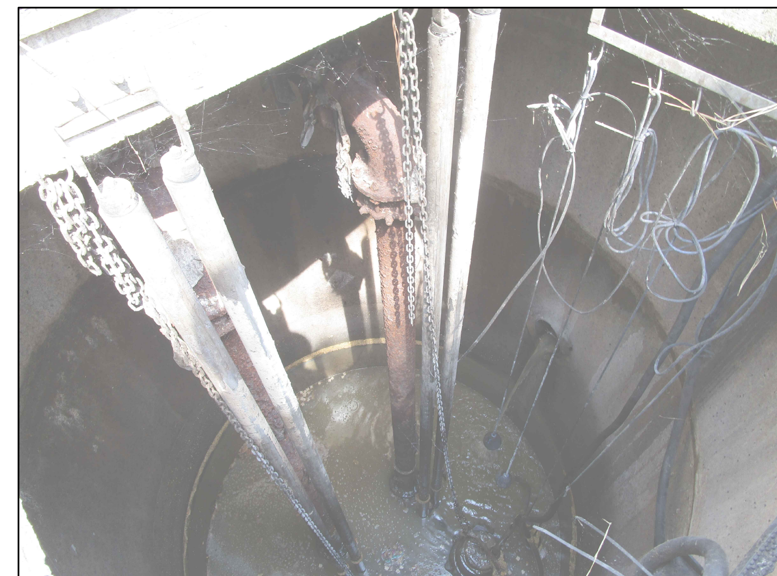
PHOTO-2 LOOKING INTO WET WELL
