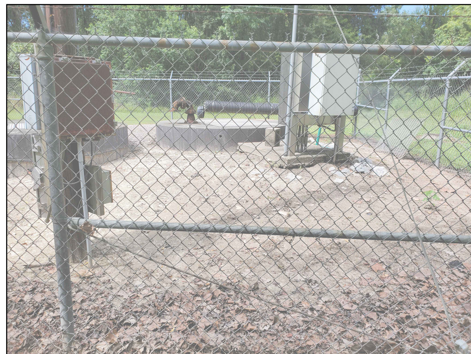
PHOTO-9 LOOKING NORTH
