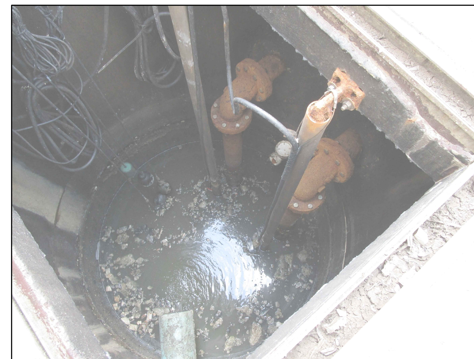
PHOTO-2 LOOKING INTO WET WELL
