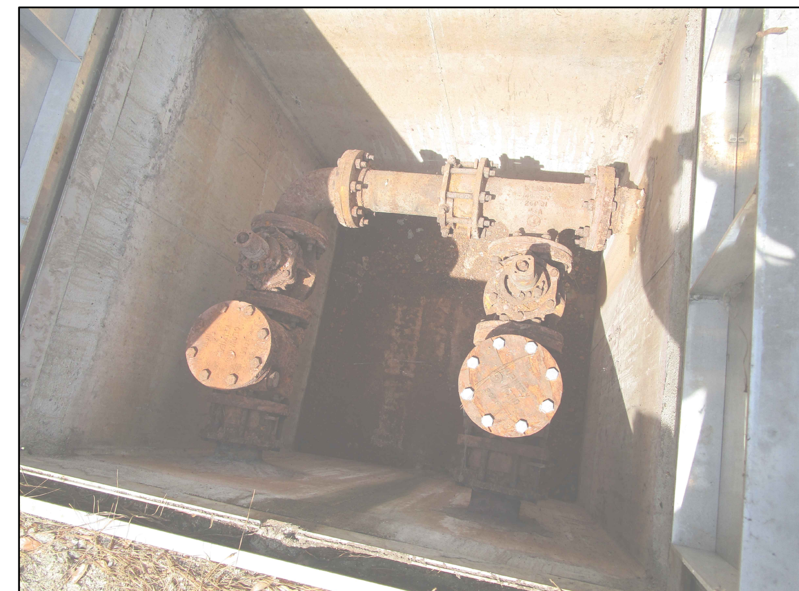
PHOTO-3 LOOKING INTO VALVE VAULT
