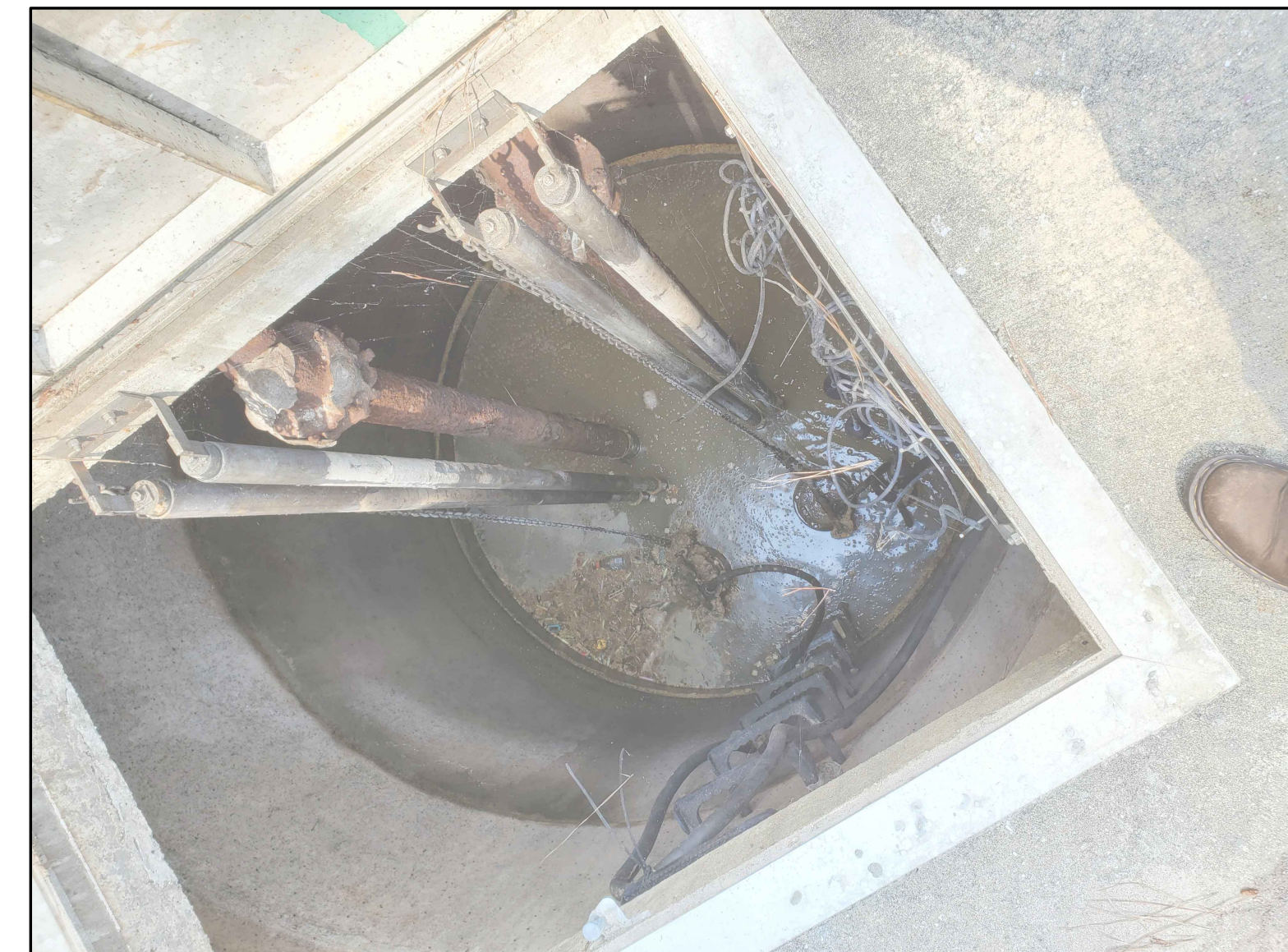
PHOTO-1 LOOKING INTO WET WELL
