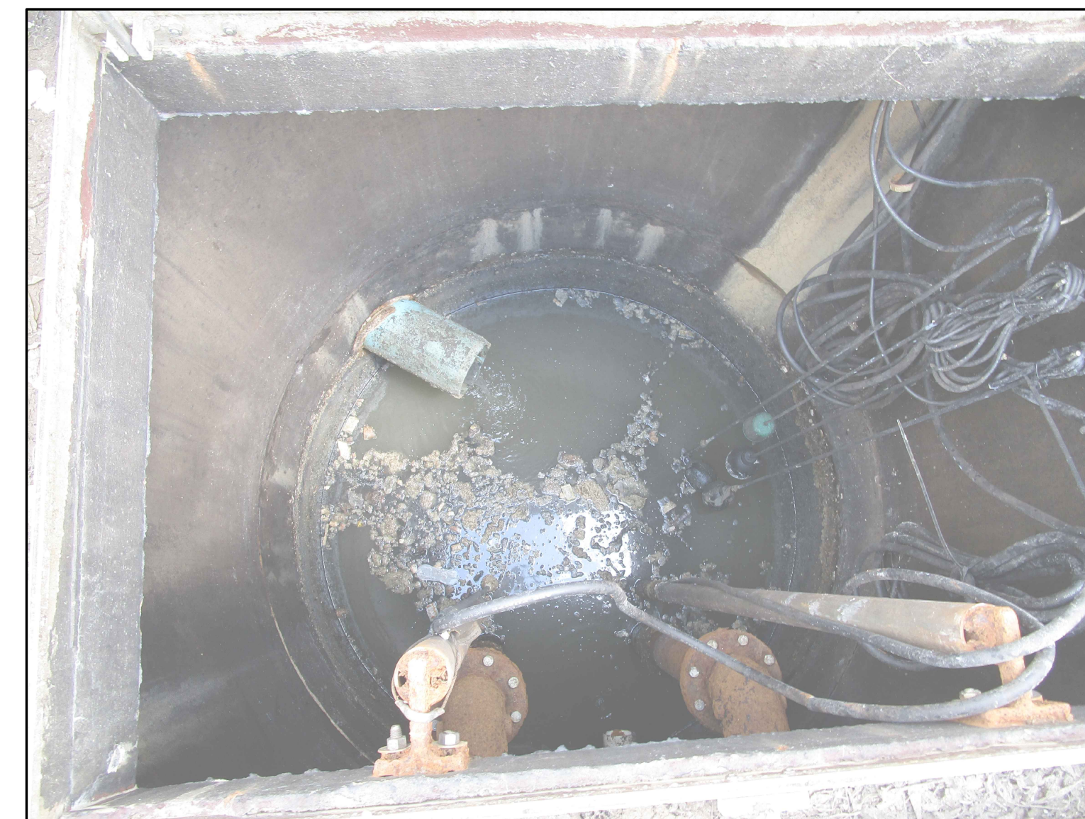
PHOTO-1 LOOKING INTO WET WELL
