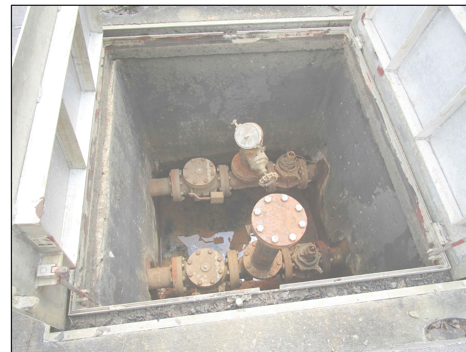
PHOTO-3 LOOKING INTO VALVE VAULT
