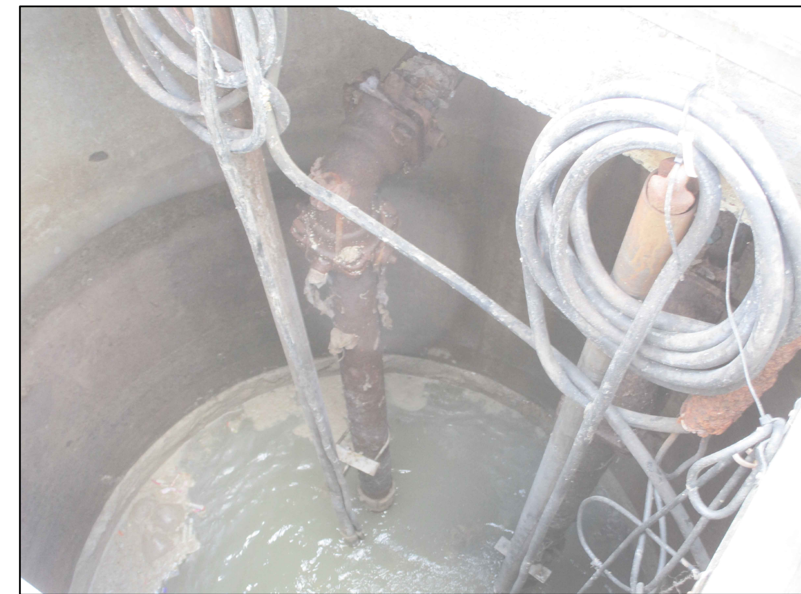
PHOTO-2 LOOKING INTO WET WELL
