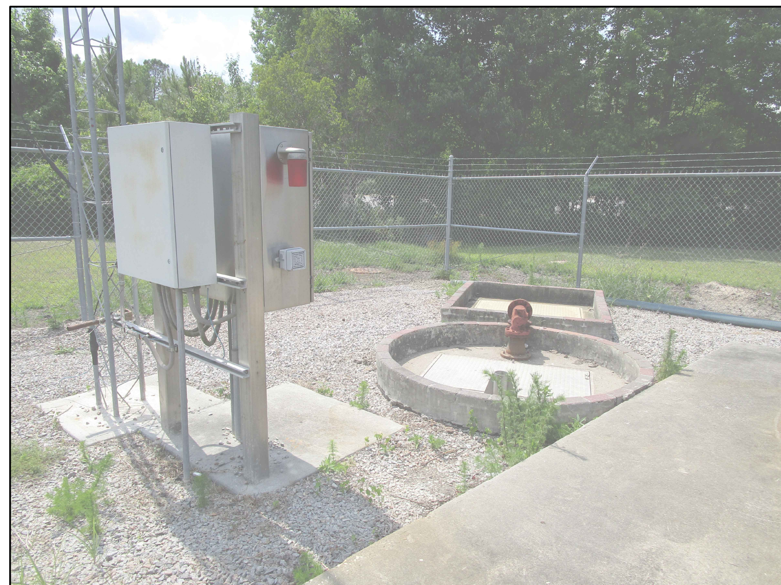
PHOTO-8 LOOKING NORTHWEST AT PUMP STATION AREA OF SITE
