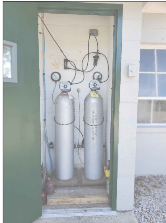
PHOTO 3 - LOOKING SOUTH TOWARD CHLORINE GAS ROOM
