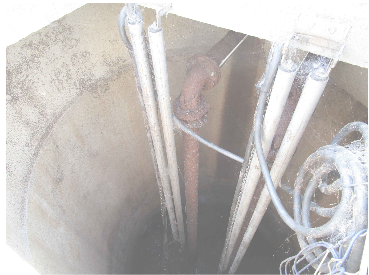
PHOTO-2 LOOKING DOWN INTO WET WELL
