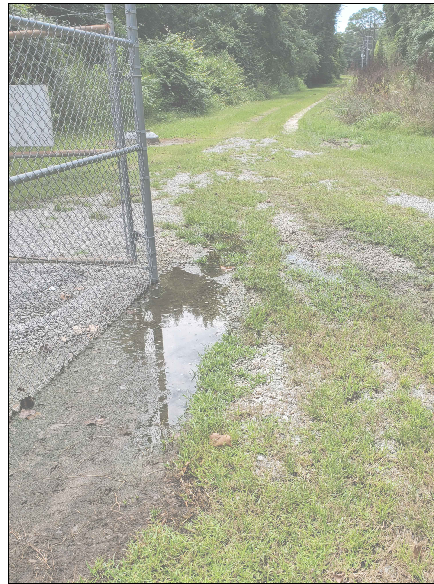
PHOTO-10 LOOKING WEST TOWARD ACCESS ROAD FROM PUMP STATION SITE
