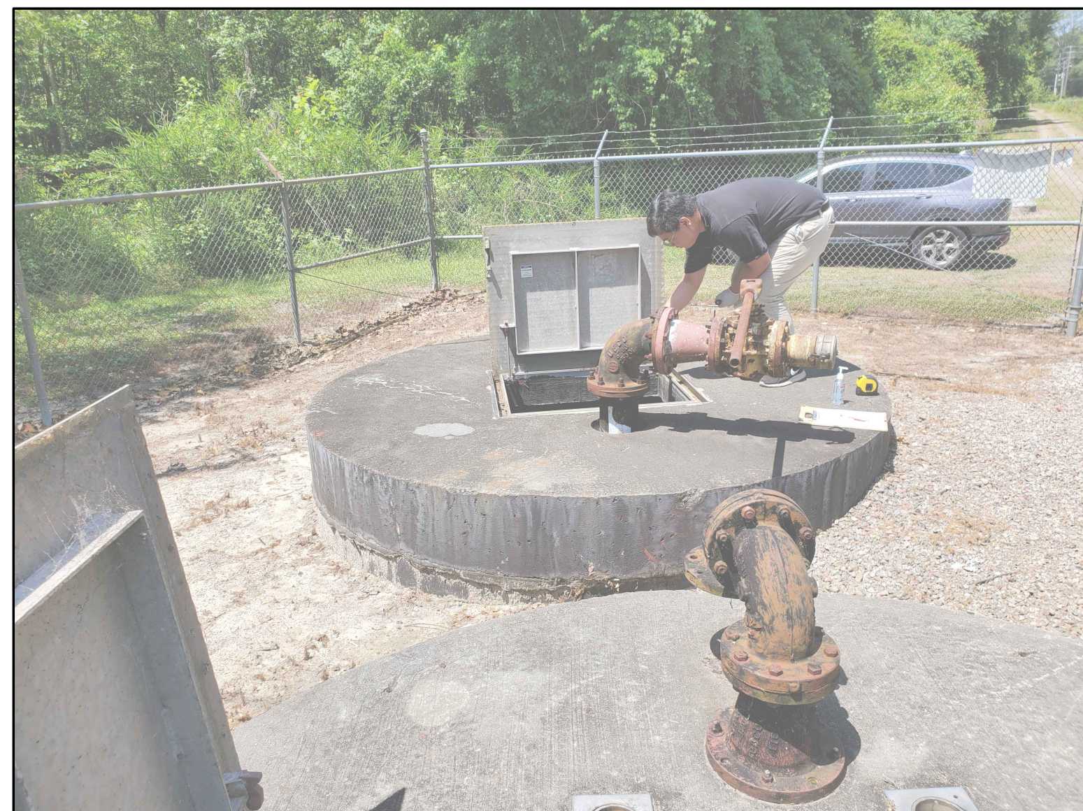
PHOTO-8 LOOKING SOUTHWEST FROM WET WELL TO VALVE VAULT
