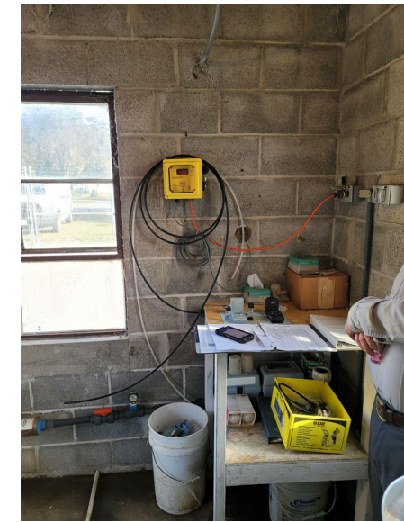
EXISTING INTERIOR LOOKING NORTH
