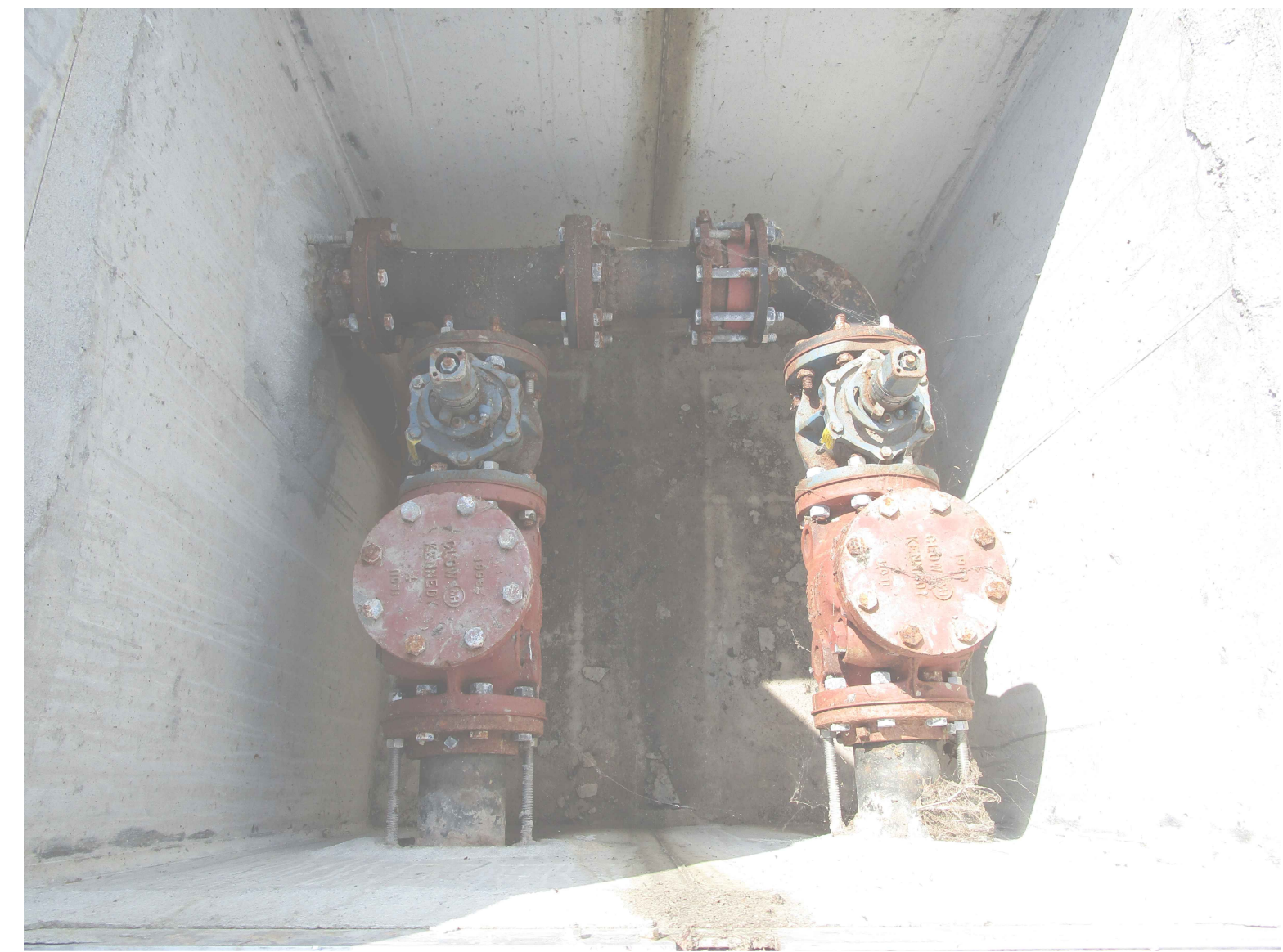
PHOTO-3 LOOKING DOWN INTO VALVE VAULT
