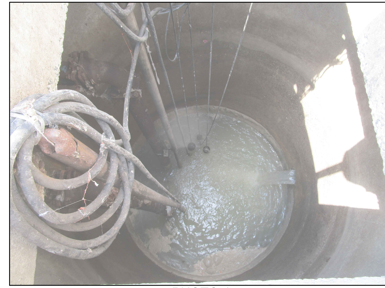
PHOTO-1 LOOKING INTO WET WELL
