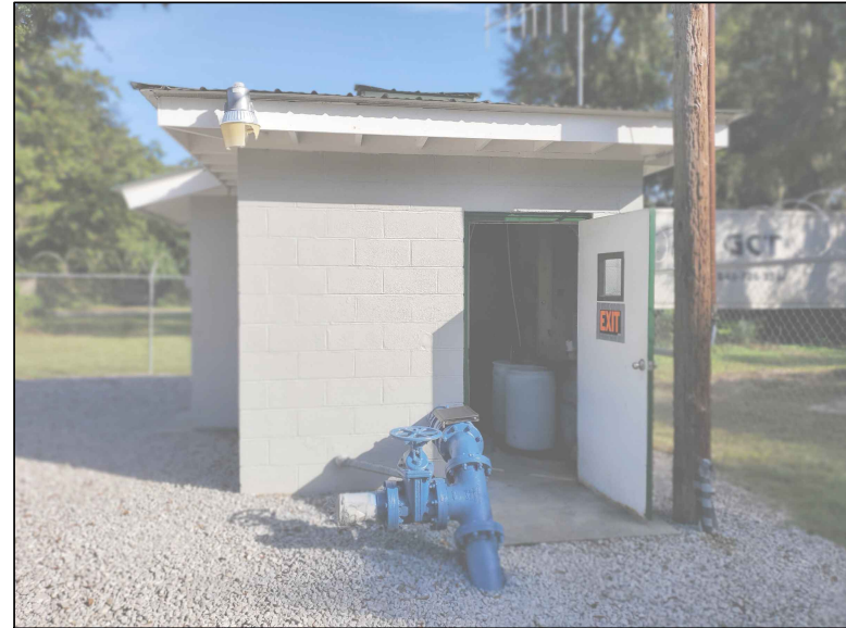
PHOTO 1: LOOKING EAST TOWARD WELL BUILDING
