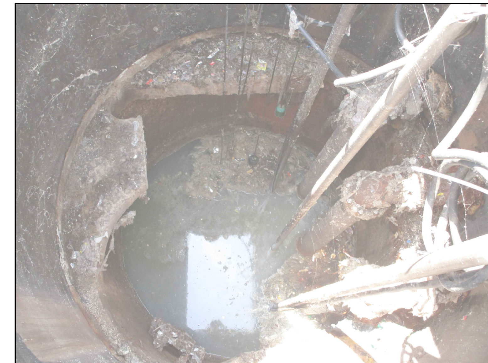
PHOTO-1 LOOKING DOWN IN WET WELL
