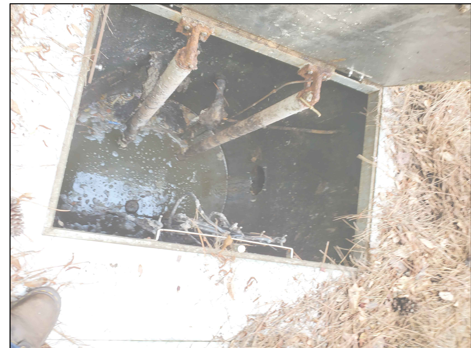
PHOTO-9 LOOKING WEST AT WET WELL
