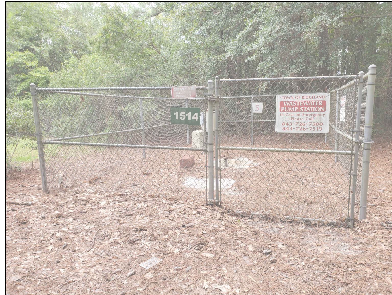
PHOTO-5 LOOKING EAST AT PS-5
