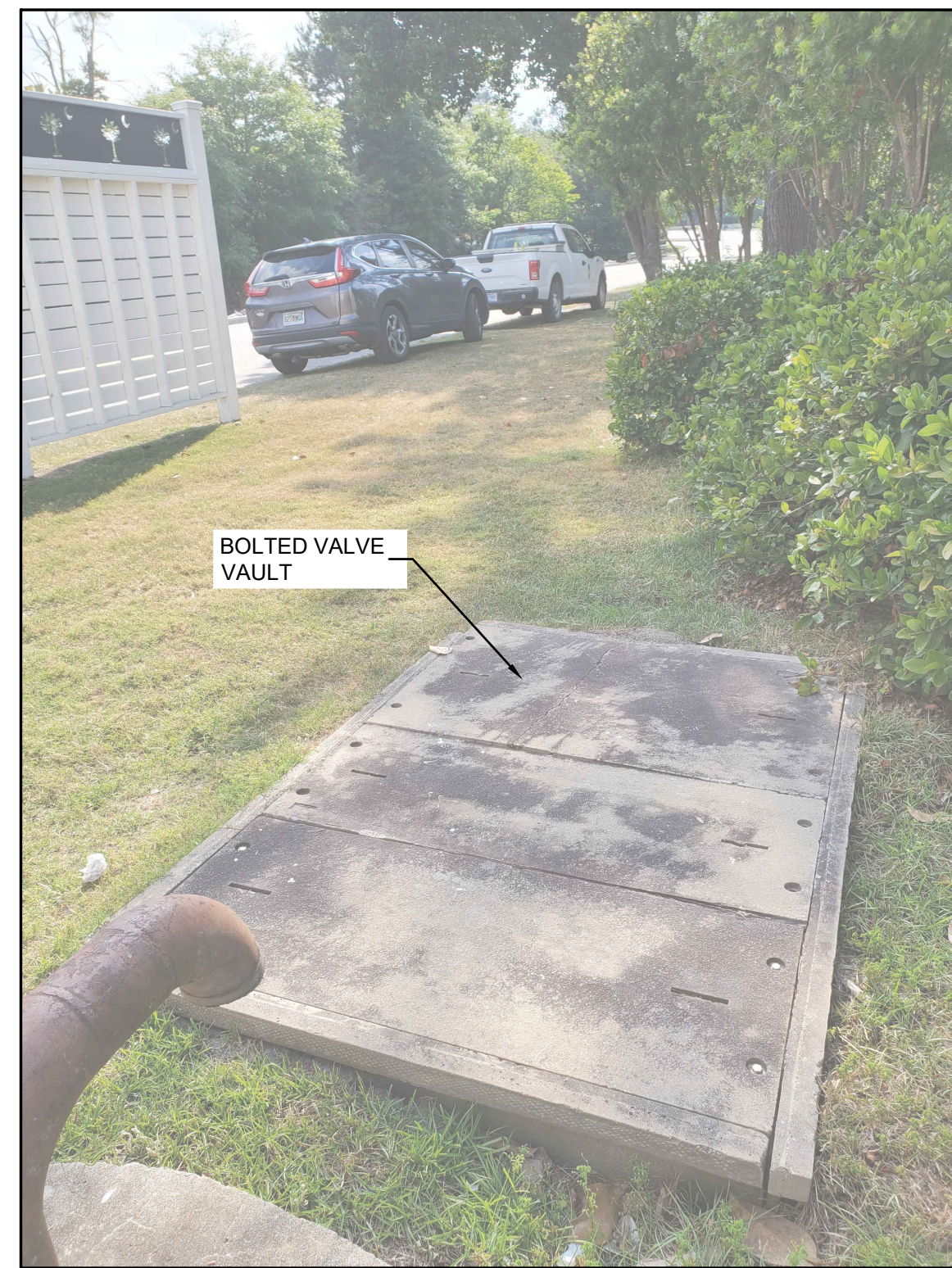
PHOTO-7 LOOKING WEST OVER VALVE VAULT
