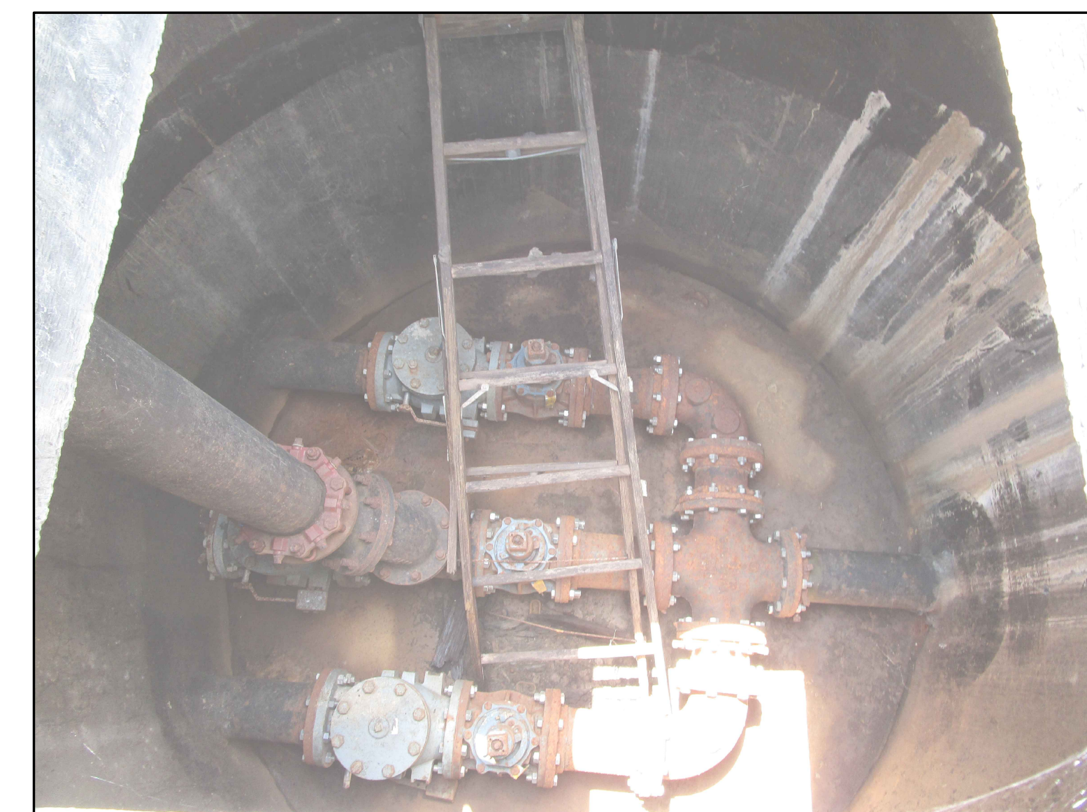
PHOTO-3 LOOKING DOWN IN VALVE VAULT
