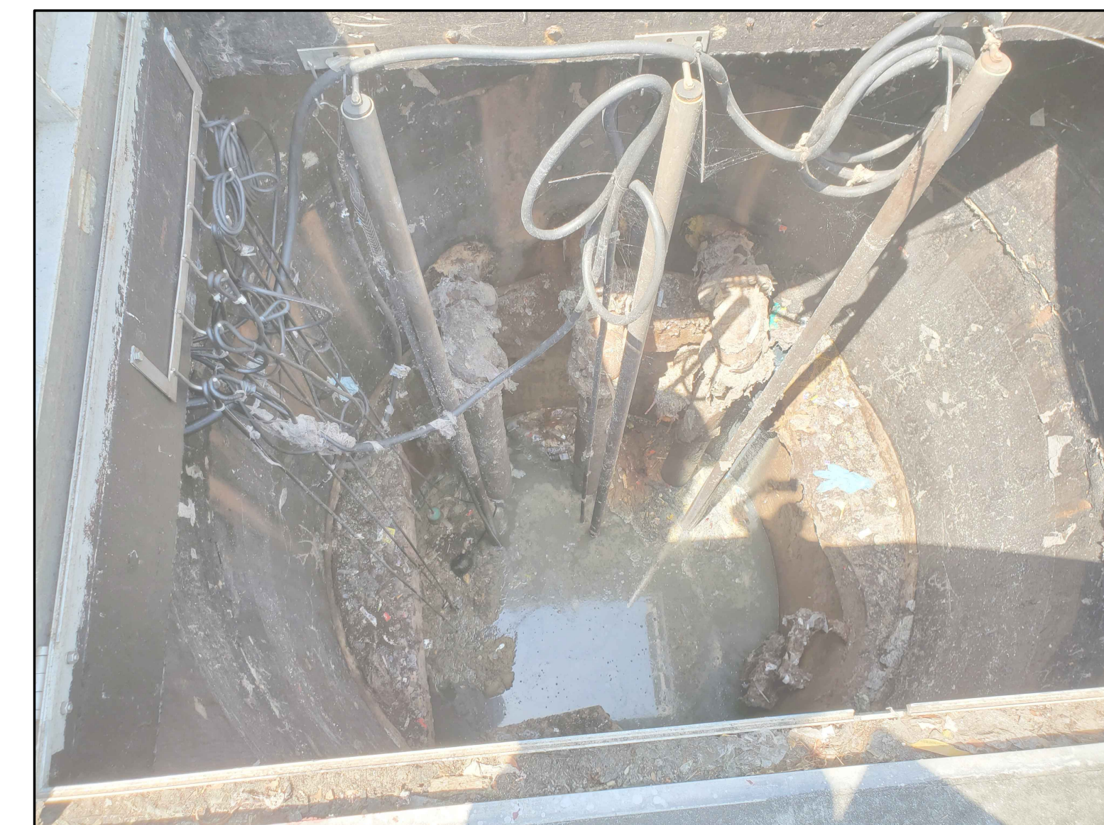
PHOTO-2 LOOKING DOWN IN WET WELL
