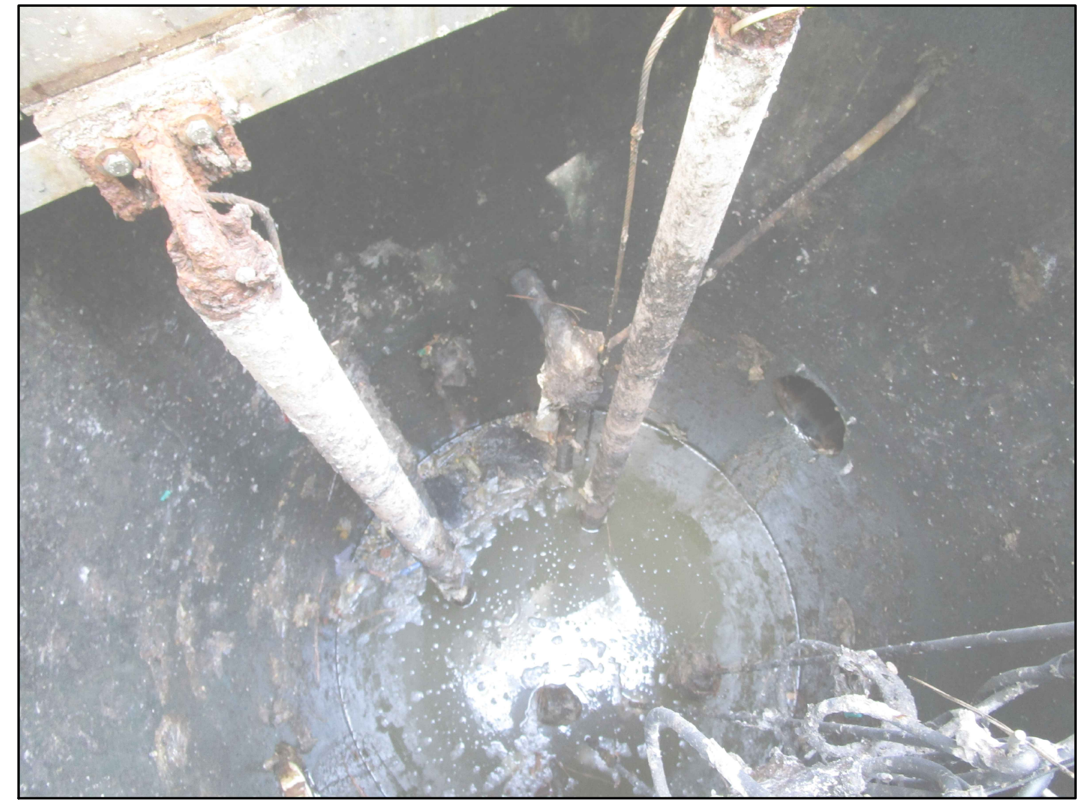
PHOTO-1 LOOKING INTO WET WELL
